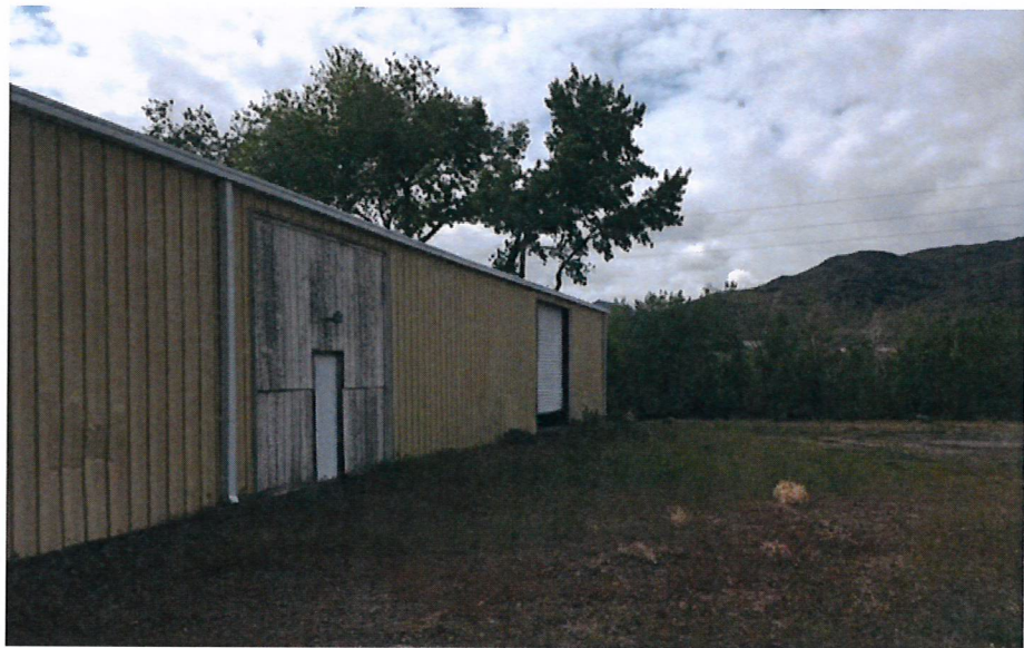
Existing industrial building
